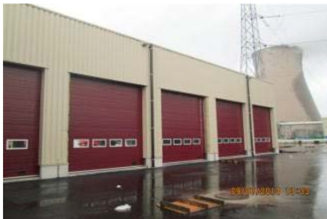
Figure 7: Construction completed of the new storage building at Doel NPP.
